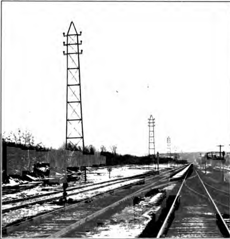
FIG. 82.—Flexible steel tower line.
